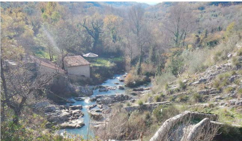
Fig. 4.21. Sant' Angelo a Fasanella, old mill.
