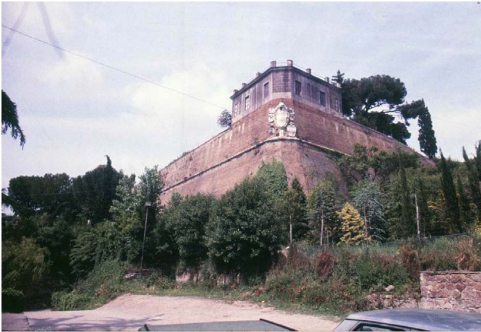
Fig. 1. General view of the bastion in its environment. Photo by C.B. 1986.
