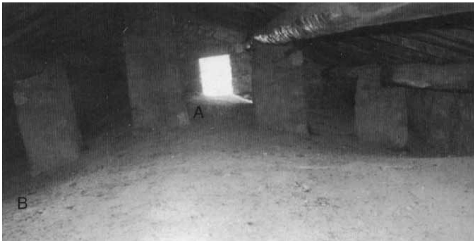
Fig. 25. Santa Maria Assunta, detail of the extradosed vault.
