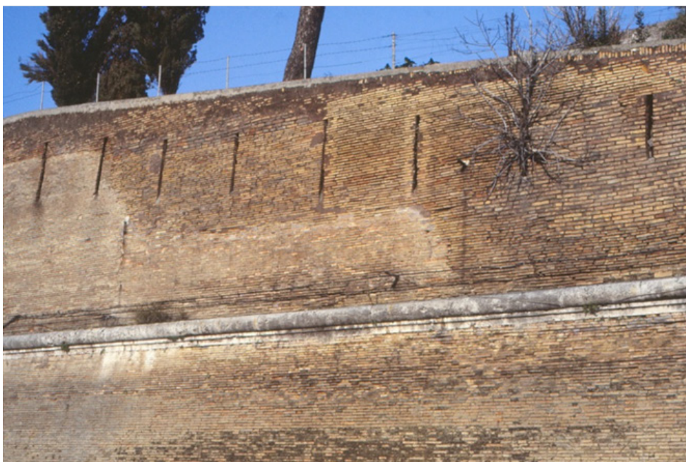
Fig. 21. Detail of the toro and the loopholes. Photo by C.B. 1985.
