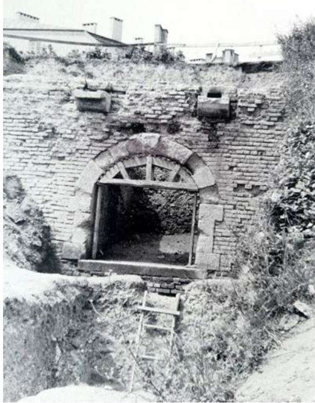
Fig. 37. Works in progress on the perimeter of the bastion of the city. Photo by C.B., July 1983.
