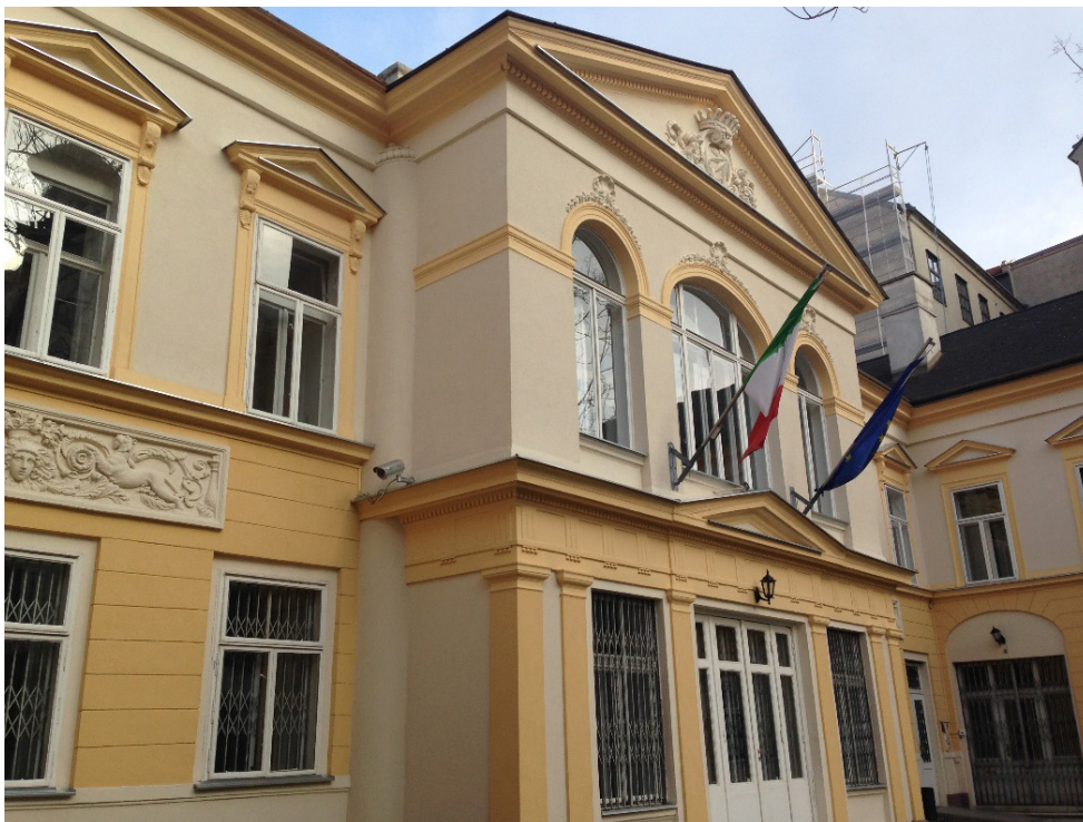
Fig. 18. Intervention of treatment of surfaces and protection of the cornices (2014-2015). Photo by Paola Zofrea.
