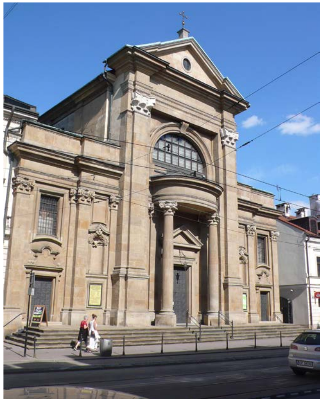
Fig. 16. Cracow, Church of the Missionaries. The façade after a new surface treatment. Photo by C.B., June 2019.
