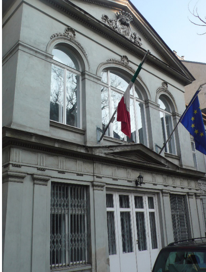
Fig. 17. Palazzo Sternberg, façade before restoration. Photo by C.B. 2014.
