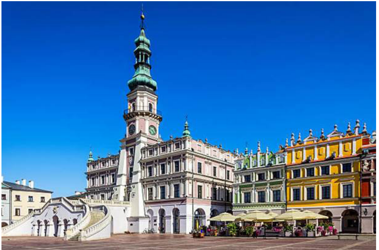
Fig. 33. Market Square with the City Hall, before and after the restoration interventions. Photo by C.B., November 1981 and 2015.
