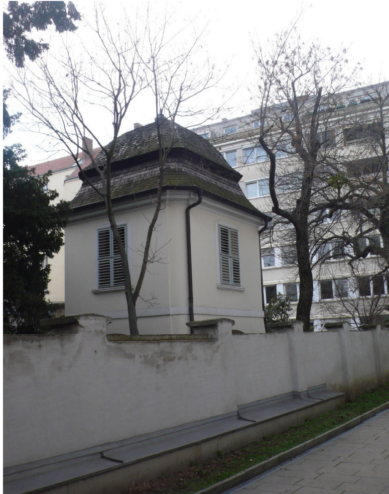
Fig. 8. Gartenpavillon , partial view of the first floor and of crowning element. Photo by C.B. 2016.
