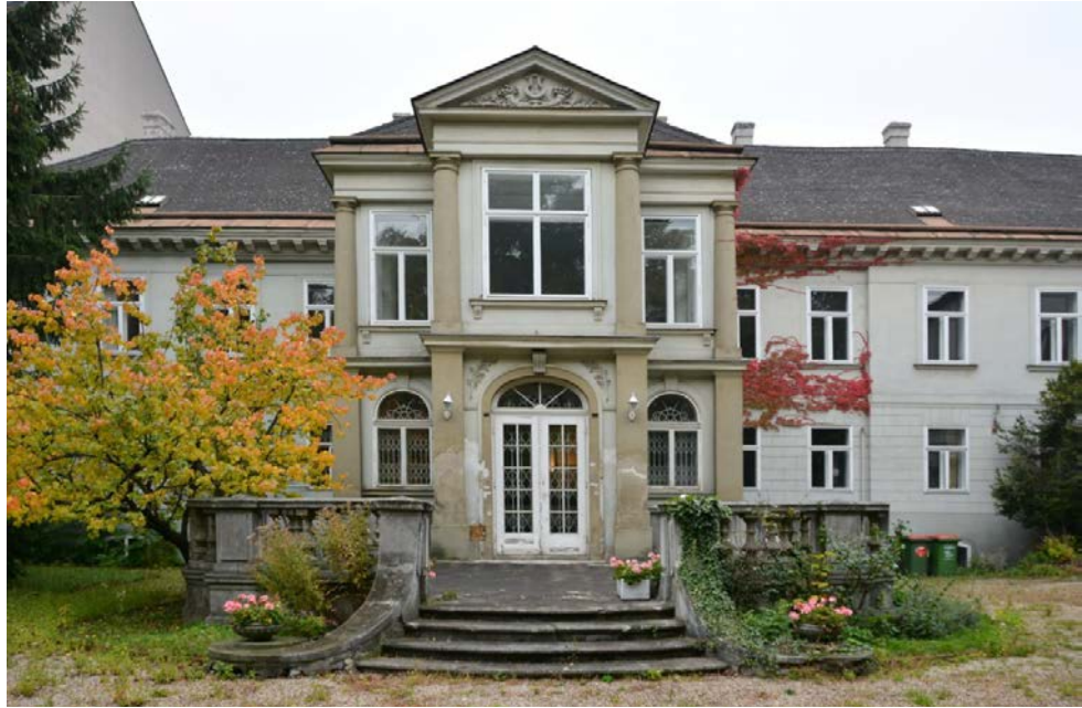
Fig. 19. Palazzo Sternberg, façade before restoration. Photo by C.B. 2014.
