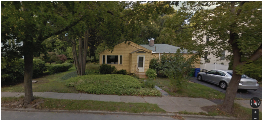
Figure 1: Hartman Road House, Google Maps Image Capture: September 2013.
