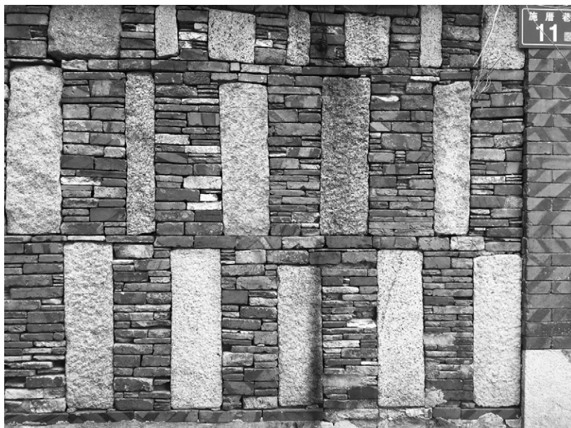
Xi'ancun, City of Anhai, Local construction techniques. Mixed stone and brick masonry.
