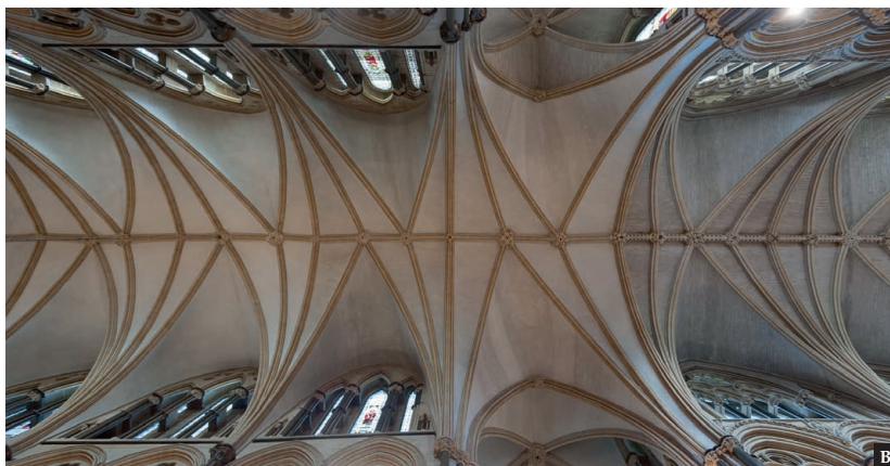
Figure 2.2. Cross vaults forms: [A] diagrammatic plan of Central European and English Gothic vaults after (Wilson, 1990) and [B] the so-called crazy vaults in the St. Hugh's Choir of the Lincoln Cathedral, UK ©John Reynolds
