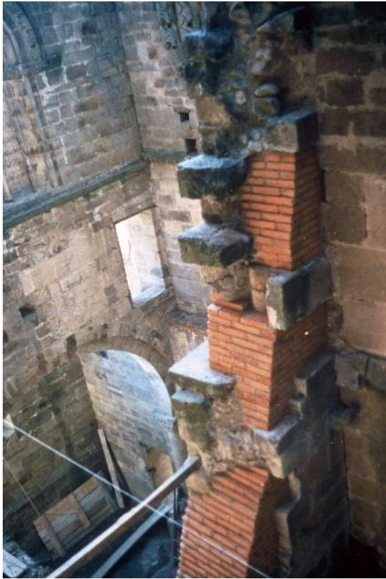
Fig. 38. Buttress, Carracedo Monastery, León, 1990. Restoration by S.P. Arroyo and Susana Mora.
