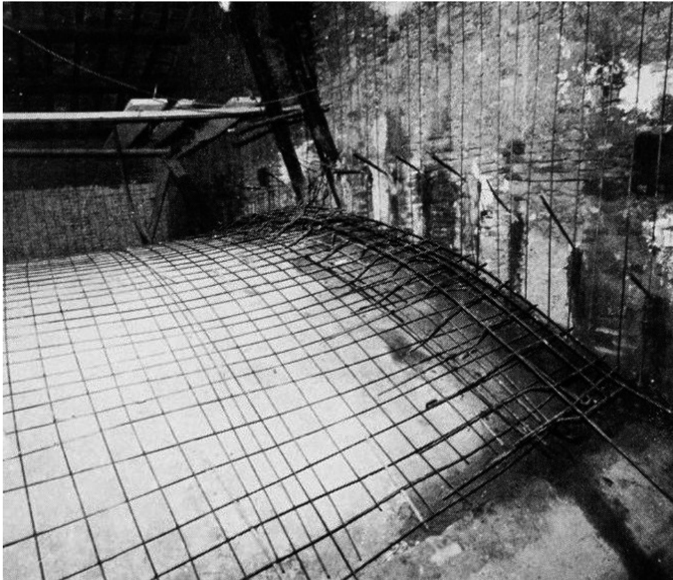
Fig. 22. San Silvestro in Capite, Roma. F. Lizzi Method. From F. Lizzi, The static restoration of monuments , Sagep Publisher, Genova 1982, p. 24.
