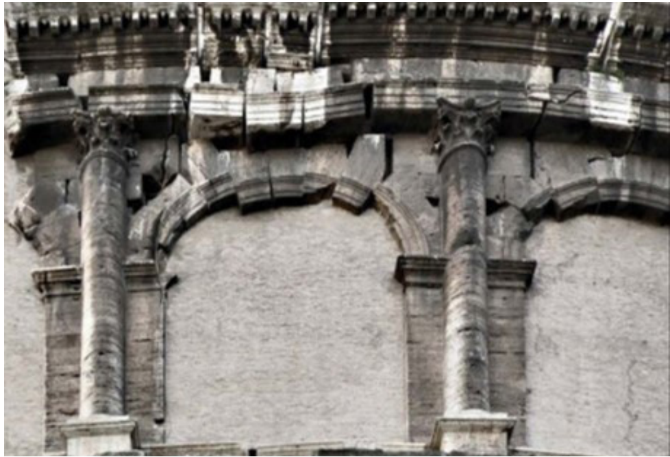
Fig. 3. Colosseo . Diagnose of the construction (physical approach). Photo by Susana Mora, 2010.
