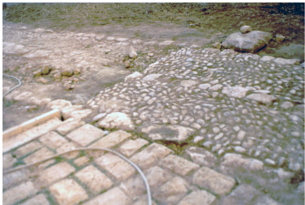
Fig. 9. Church of Santa María de Los Reyes. Grijalba. Burgos. Exterior paving. Photo by Susana Mora.
