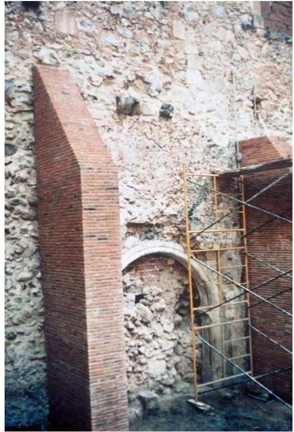
Fig. 39. Buttress, S.P. de Arlanza, Burgos, 1989. Restoration by S.P. Arroyo and Susana Mora.
