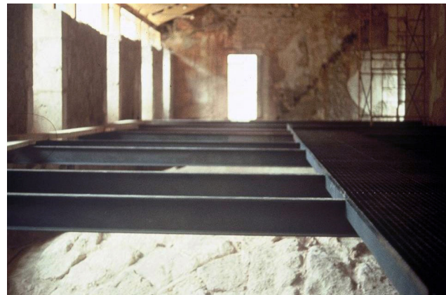
Fig. 20. New beams anchors in the vaults of the Refectory, San Pedro de Arlanza, Salvador Pérez Arroyo and Susana Mora. Photo by Susana Mora, Burgos, 2012.
