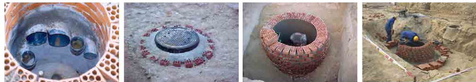
Fig. 55. Circular drainage well. Photos by Celia Barahona.
