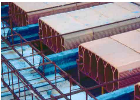
Fig. 20. On the left: Placement of in-floor bricks and compression reinforcement of joists. On the right: Openings. Photos by Fernando Ripollés and Celia Barahona.
