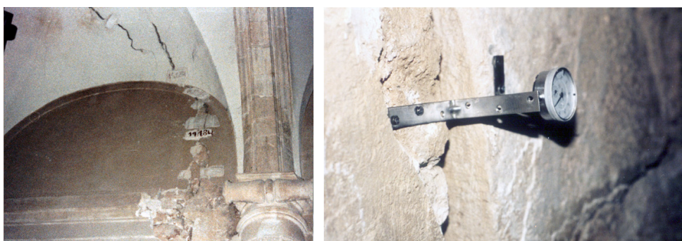
Fig. 43. San Bartolomé Parish Church. Structural consolidation. Foundation reinforcement through micropiles. Sewed of factories. Follow-up through instrumentation. Susana Mora. Tarazona de la Mancha, Albacete 2000.
