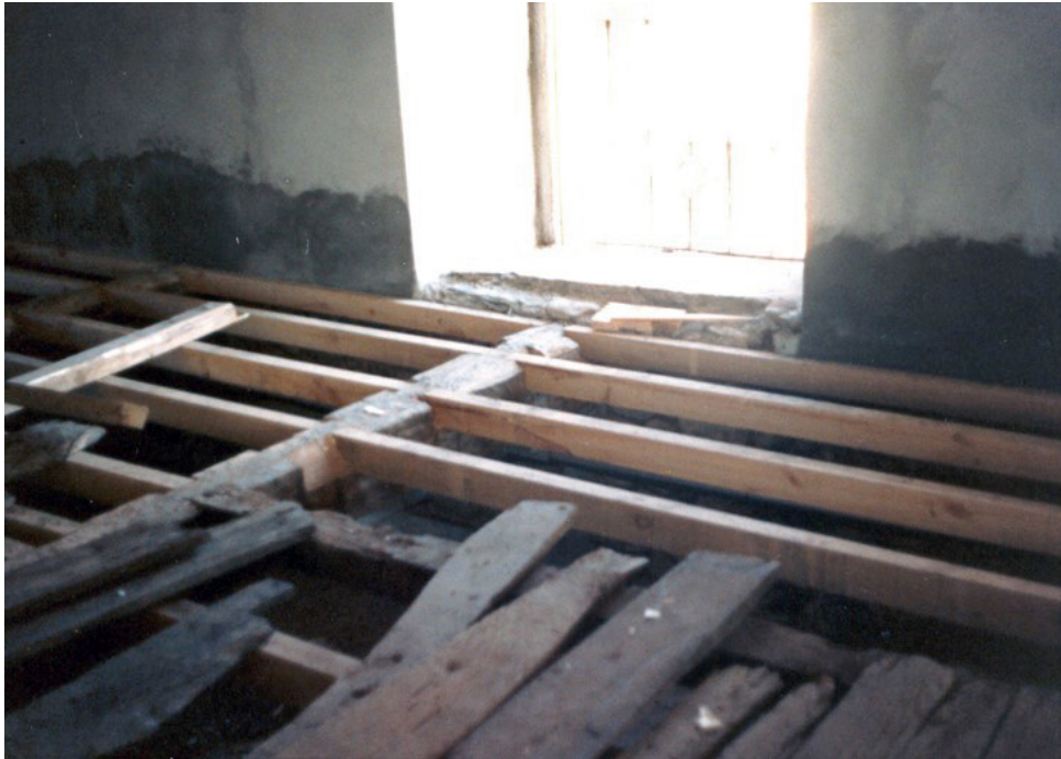
Fig. 27. Library floor reinforcement of Santa María de Carracedo Monastery. Restoration by S. Perez Arroyo and S. Mora. Photos by Susana Mora, 1990.
