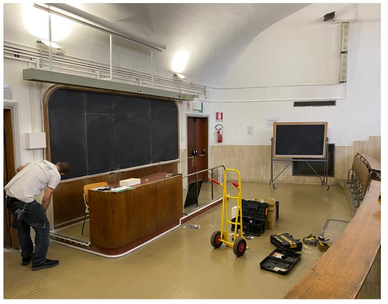
Figure 35 - The hall of the classroom tower on the first floor; note the niche over the door leading to the staircase, closed by a wall and a fire door (© Salvo 2021)
