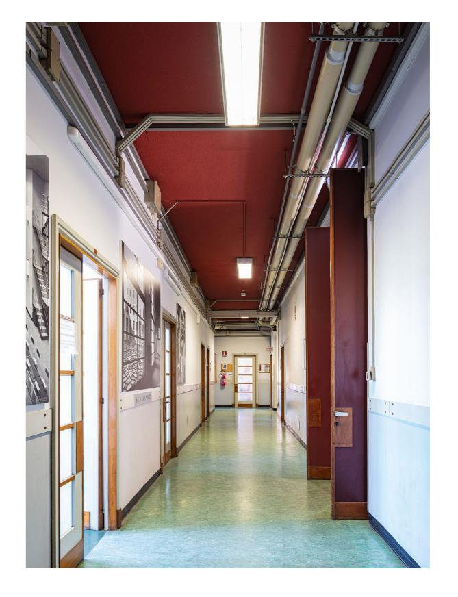
Figure 11 - Front building, first floor, bundling of cables, ducts, and wiring in the office corridor (© Sardo 2021)
