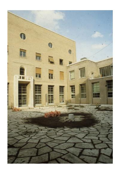
Figures 6/7 - The inner courtyard of the School of Mathematics in the mid-Eighties when the joints between the travertine slabs of the paving had just been filled with concrete (BFAR\_pht\_04, BFAR\_pht\_05)
