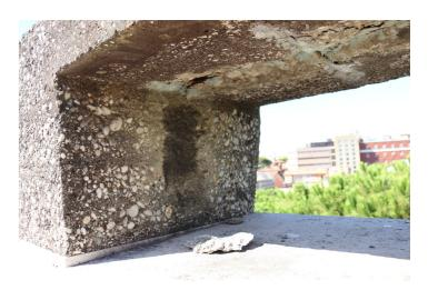
Figure 7 - Asphalt mortar integration on concrete of the crowning frame (© Santarelli, Giorgi, Ciacchella, Pandolfi 2020)
