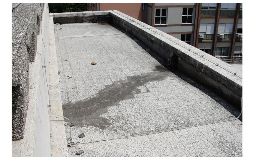
Figure 17 - Fragments of the concrete crowning frame that have fallen on the roof of the library depot (© Salvo 2011)
