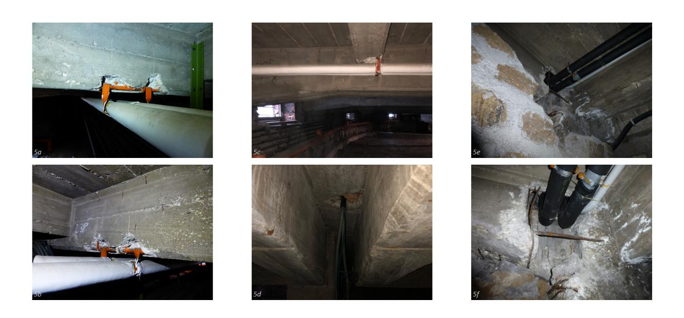
Figure 5 a/f - East curved wing, basement level: a) pipes hanging on longitudinal reinforcements (© Liberatore 2020); b) stirrup oxidation, pipes hanging on longitudinal reinforcements (© Liberatore 2020); c) stirrup oxidation, pipes hanging on longitudinal reinforcements (© Martella 2020); d) hole in the reinforced concrete slab for the passage for cables (© Martella 2020); e-f) hole in a reinforced concrete beam for the passage for pipes (© Sorrentino 2020).
