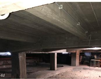
Figure 4 a/d - East curved wing, basement level: a) bars oxidation, spalling of concrete, cracks in the masonry wall (© Martella 2020); b) bars oxidation, spalling of concrete, cracks in the masonry wall (© Martella 2020); c) oxidation of stirrups and longitudinal bars and consequent spalling (© Liberatore 2020); d) oxidation of stirrups due to reduced concrete cover especially at the lower side corners (© Martella 2020).
