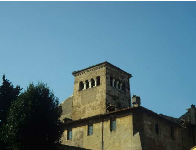
Figg. 25-26. Roma, Santi Quattro Coronati. The tower was realized during Charles the Great period and present the typical brickwork and quadrifora, and the ancient plaster, with two or three coat plaster with lime. (CB 1994)
