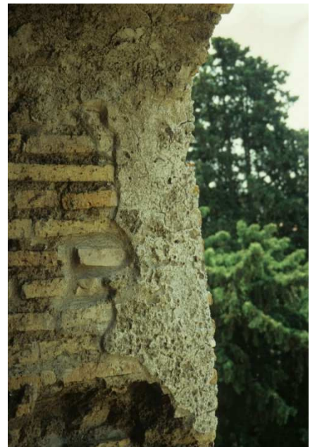
Figg. 25-26. Roma, Santi Quattro Coronati. The tower was realized during Charles the Great period and present the typical brickwork and quadrifora, and the ancient plaster, with two or three coat plaster with lime. (CB 1994)
