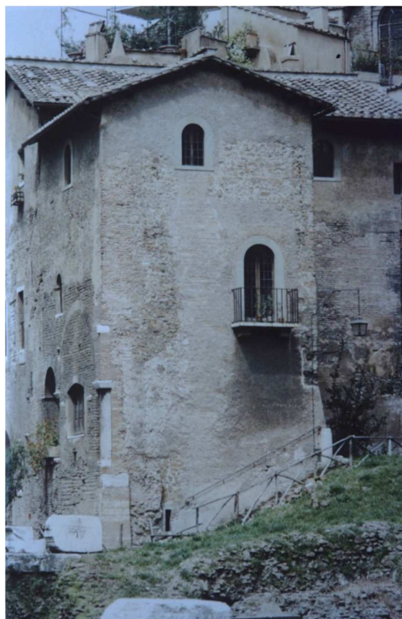
Fig. 7. Roma, medieval residences, Albergo della Catena. Example of external finishing treatment. (CB 1994)
