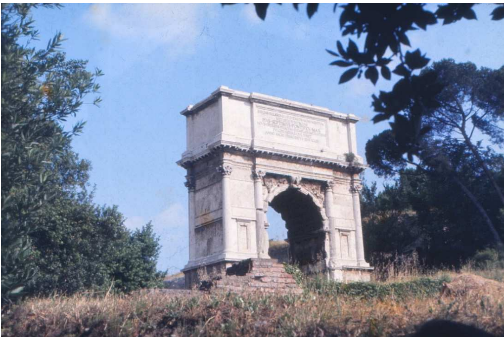
Fig. 15. Stern and Valadier "complete" the lost part in simplified form as the had suggested (1818-1824). (CB 1985)
