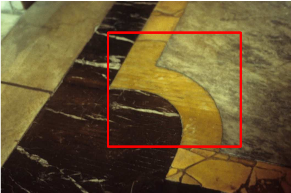
Fig. 38. Roma, Santa Barbara dei Librai, a work of Istituto Centrale del Restauro from 1983. Reintegration of the image is clear with the “ rigatino ” treatment in loss of yellow marble. (CB 1989)
