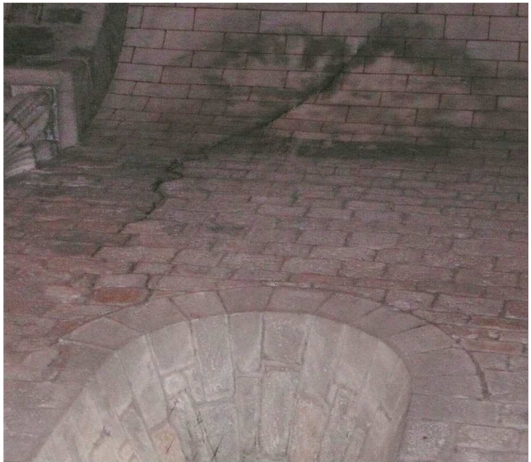
Fig. 25. Carcassonne Saint-Nazaire Cathedral, Right nave, where you can see the reintegration, separating old and new. (CB 2019)
