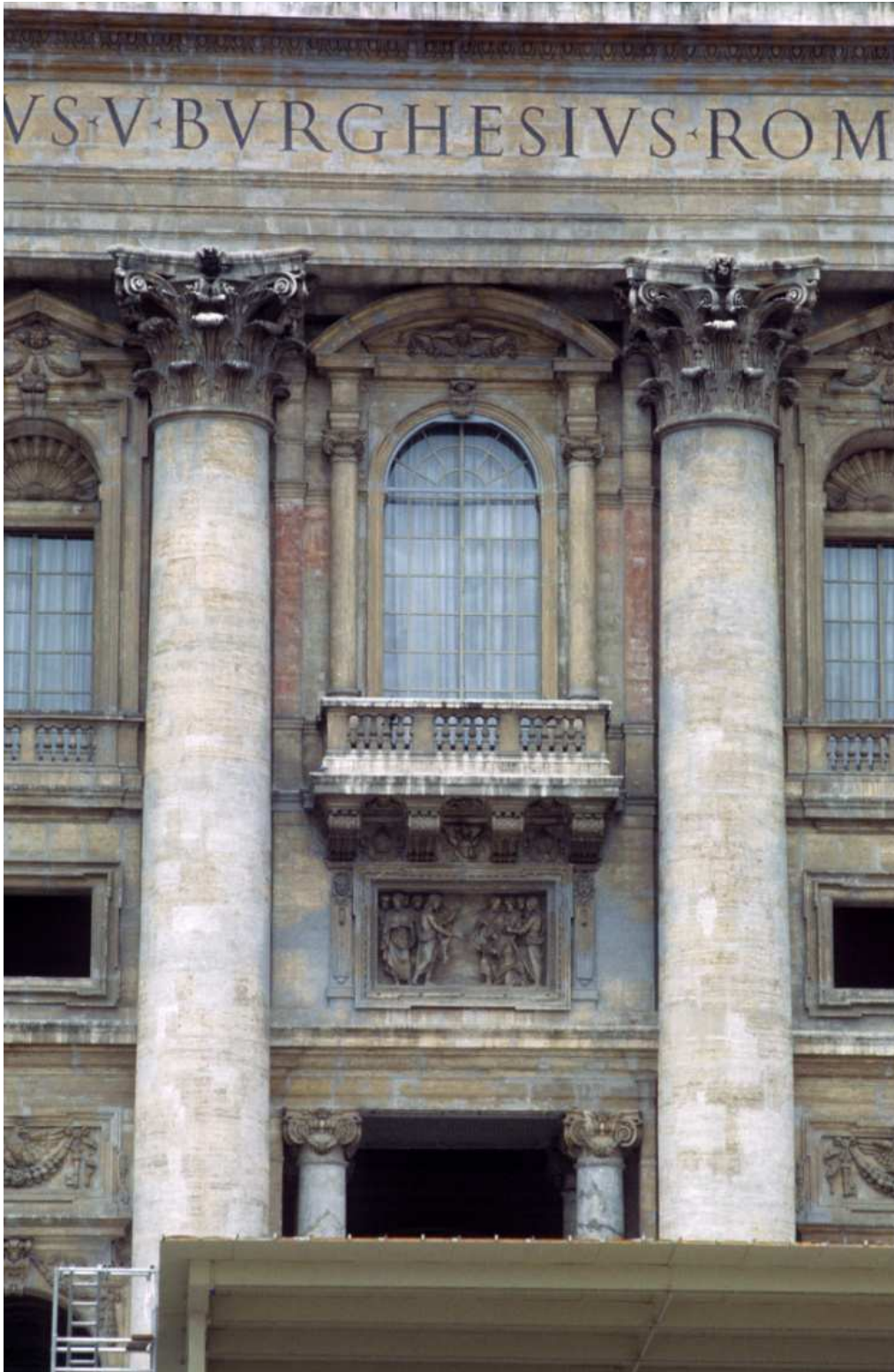
Fig. 37. Città del Vaticano, Basilica di San Pietro, Loggia delle Benedizioni. Restoration by Giuseppe Zander (1984-1986). Cleaning of the stone surface and protection. Biocide treatment and stucco applications to prevent the penetration of water in the travertine. (CB 1986)
