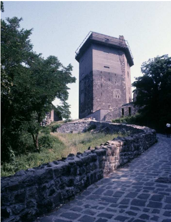
Fig. 26-27. Visegrad, Hungary, Salomon Tower. Medieval Donjon. Restoration with reinforced concrete. The theme of the reintegration of the image is clear. (CB 1980)
