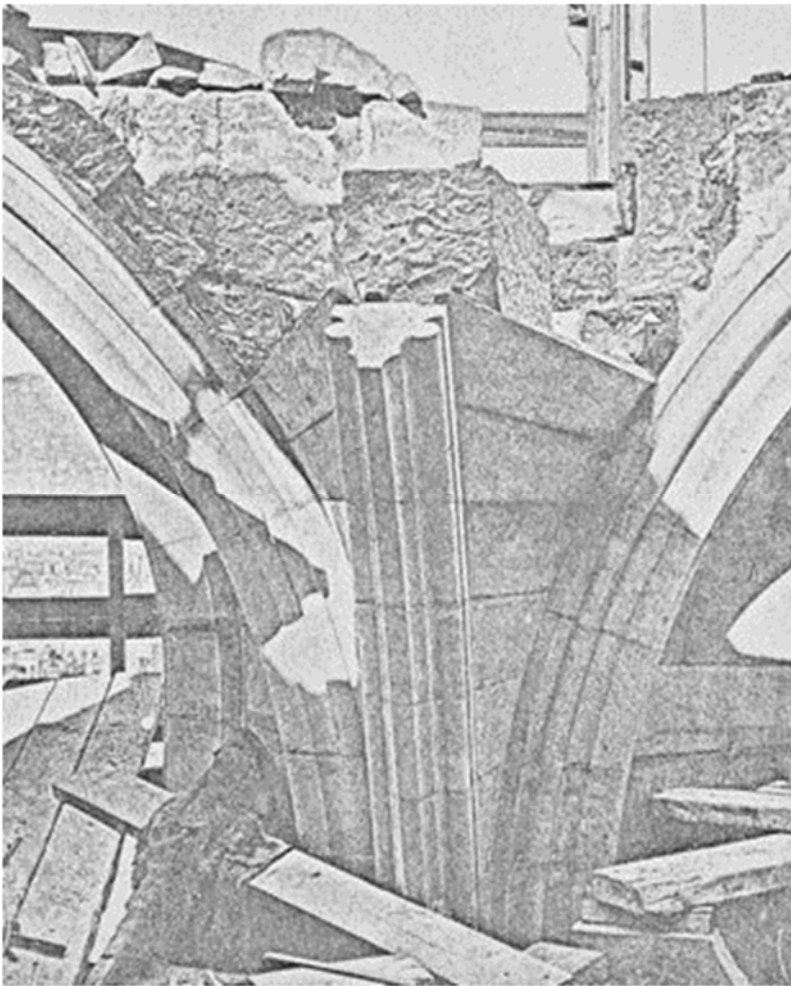
Fig. 14. Catedral de Barcelona. The construction of the new arches for the lantern.
