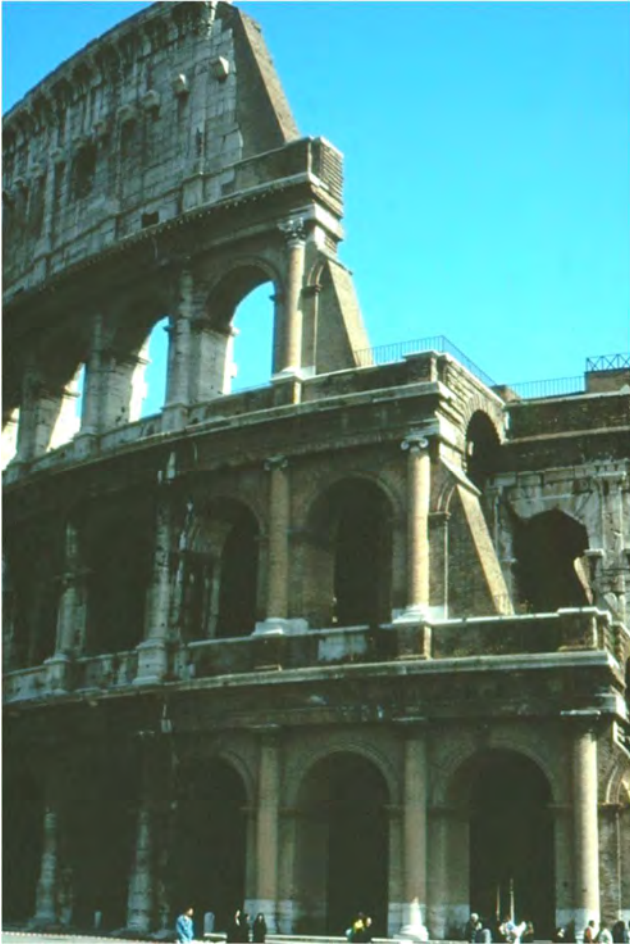
Fig. 12. Roma, Colosseo. 1824-1826: the western section was restored by Valadier, who aimed at a partial reconstitution of the architectural forms. Valadier justified the use of brick instead of stone for economic reasons. (CB 1985)
