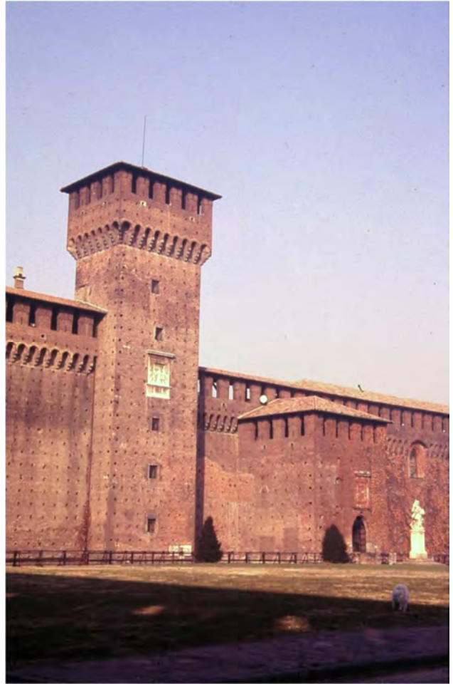
Figg. 3-4. Milano, Castello Sforzesco, the different red bricks help the comprehension of the historic restoration. (CB 1990)
