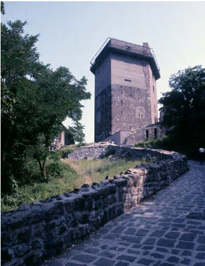
Figg. 26-27. Visegrad, Hungary, Salomon Tower. Medieval Donjon. Restoration with reinforced concrete. The theme of the reintegration of the image is clear. (CB 1980)
