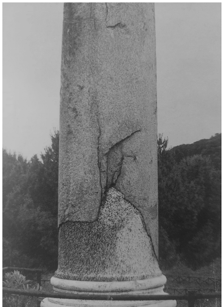
Fig. 16. Roma, Temple of Venere and Roma. Detail of a column with reintegration. (CB 1995)
