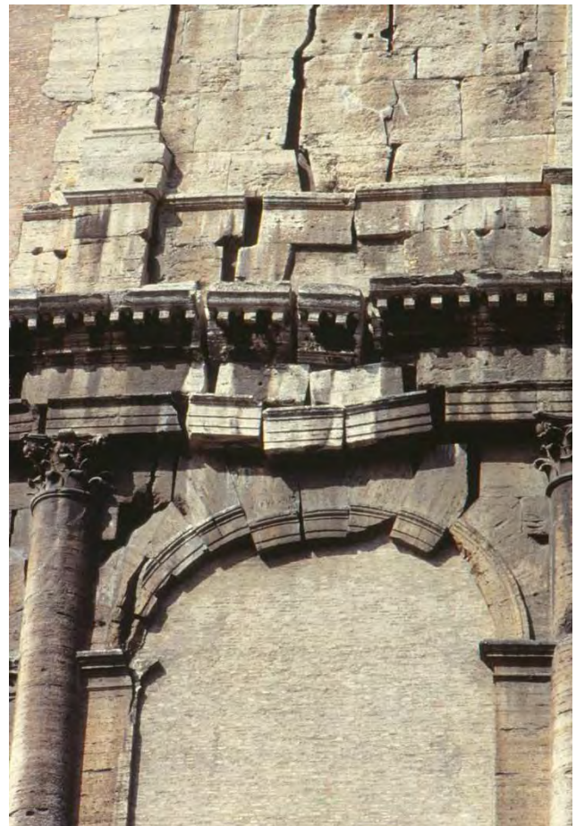
Fig. 11. Roma, Colosseo. Detail of crash moment of the arc and "architrave". (CB 1985)
