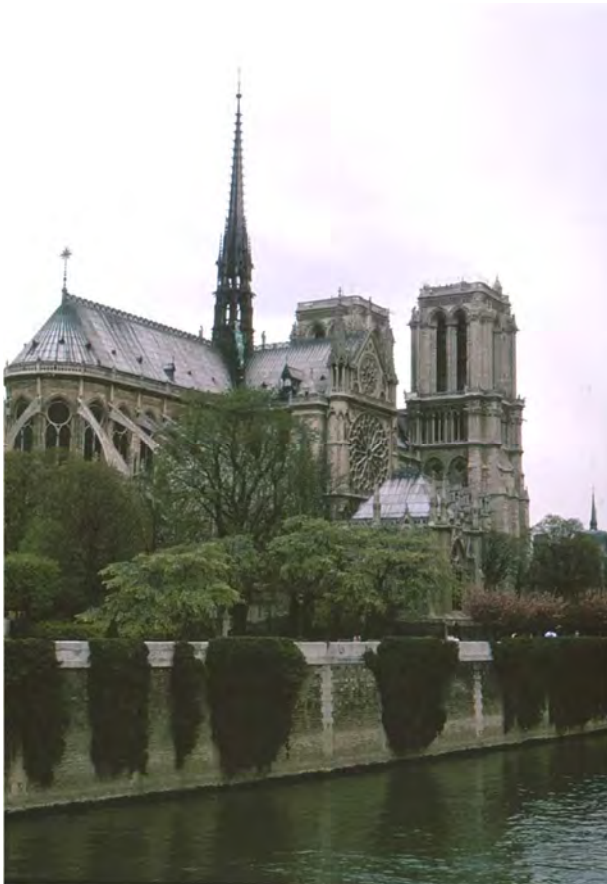
Fig. 11. Paris, Notre-Dame, the spire rebuilt with a wooden structure lead coated by Viollet-le-Duc. (CB 1983)
