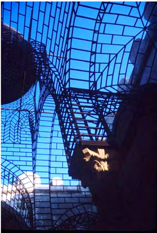
Figg. 19-20. Mazara del Vallo, San Nicolò Regale. Restoration project by Franco Minissi, reintegration of image. A slim metal structure for a new reintegration walling. The plastic materials used is perspex laminate from factory Imperial Chemical Industries. (CB 1981)
