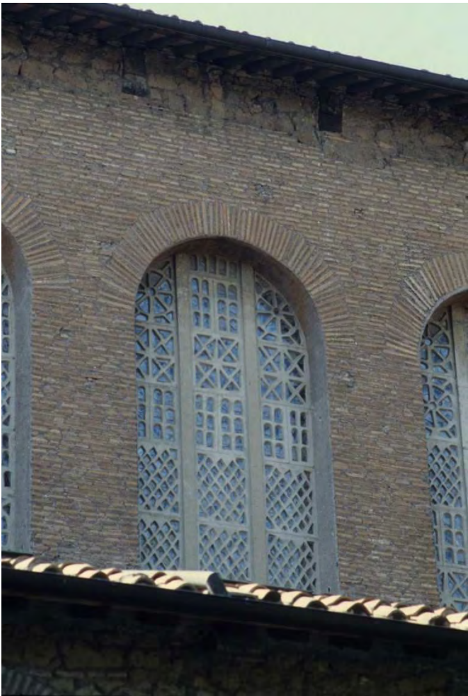
Fig. 44. Roma, Church of Santa Sabina, detail of windows with selenite barriers. (CB 1994)
