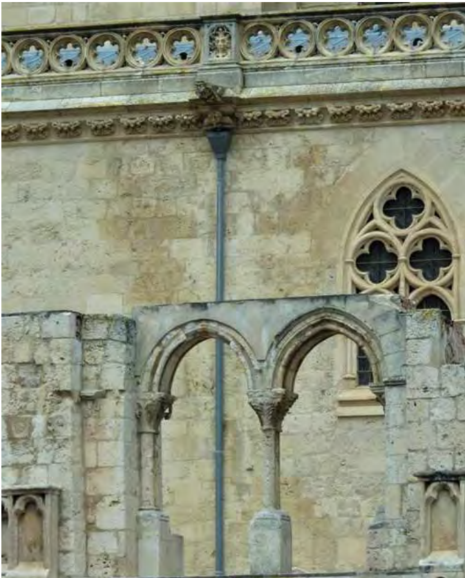
Fig. 4. Detailed image of the current state of the double window found in the demolition of 1914 and preserved by Lampérez.
