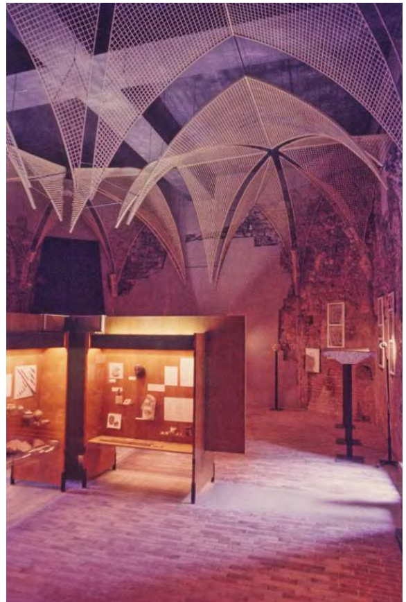
Figg. 26-27. Visegrad, Hungary, Salomon Tower. Medieval Donjon. Restoration with reinforced concrete. The theme of the reintegration of the image is clear. (CB 1980)
