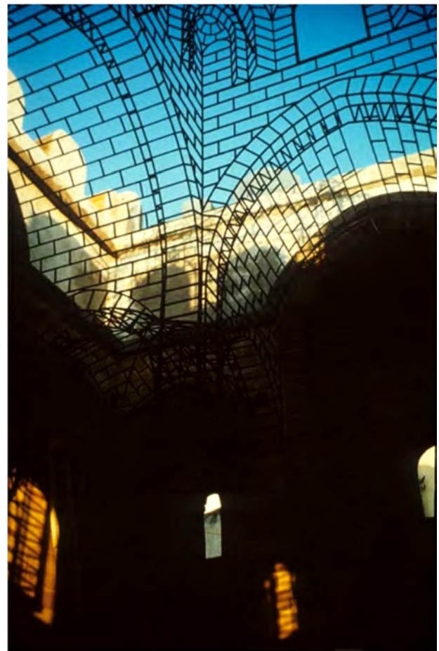
Figg. 19-20. Mazara del Vallo, San Nicolò Regale. Restoration project by Franco Minissi, reintegration of image. A slim metal structure for a new reintegration walling. The plastic materials used is perspex laminate from factory Imperial Chemical Industries. (CB 1981)
