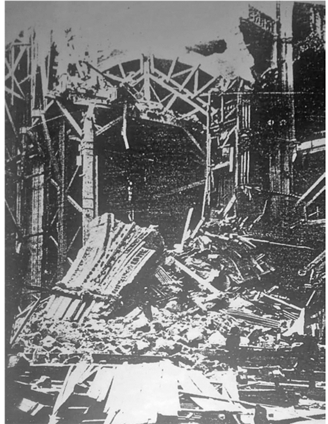
Fig. 7. Catedral de Sevilla. The southwest corner pillar collapse. 1st august 1888.
