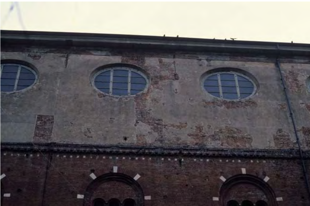
Fig. 35. Milano, Palazzo della Ragione (1978-1982). Surface treatment. The conservation project and the direction of the works has been done by Marco Dezzi Bardeschi. The consolidation of the surface and the wooden windows, without making disappear the history, but including some functional detail when are necessities. (CB 1989)
