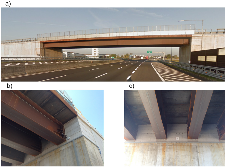
Fig. 3.1. Integral abutment bridge which inspires the case study: (a) general view of the bridge, (b) detail of the integral connection at abutment-deck node, (c) detail of four welded I-shaped plate girders.
