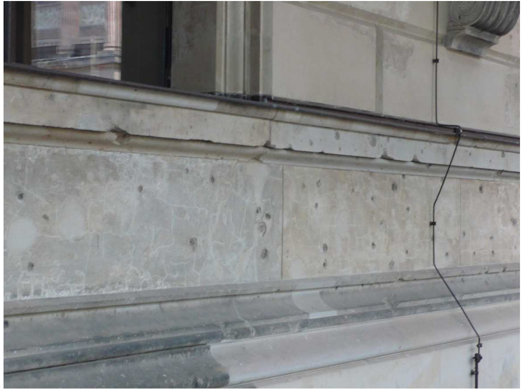
Fig. 13 - Reintegration with pieces of different types of stone. The War drama has been preserved. (CB 2009)
