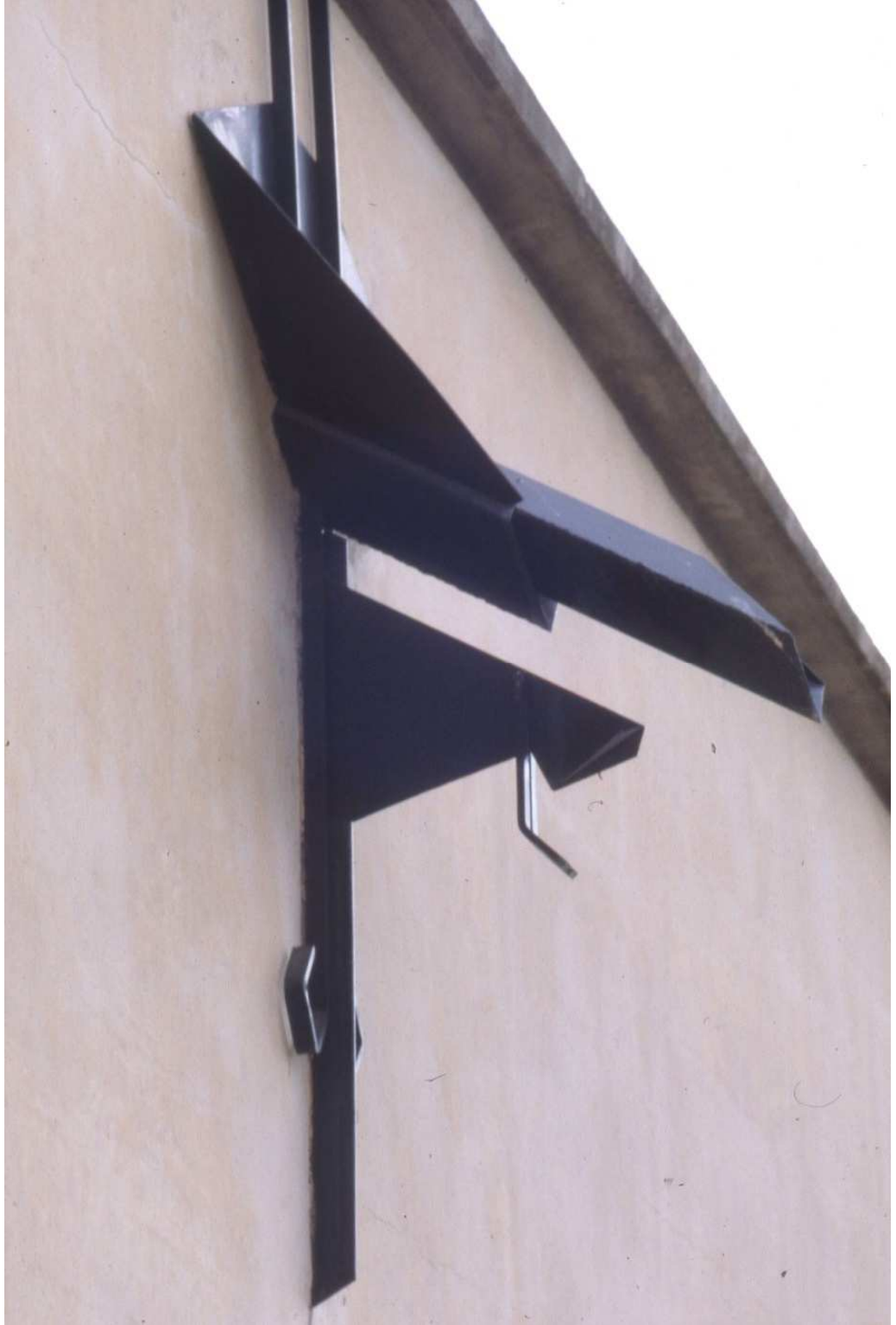
Fig. 5 - Particular for rainwater drainage in Agrigento. (CB 1982)
