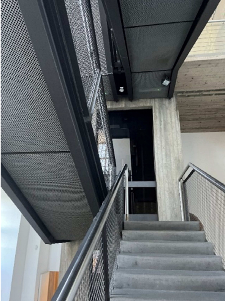
Fig. 16 - Staircases and elevator. (CAL 2023)
