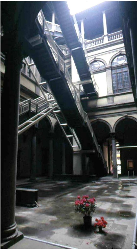
Fig. 26 - Firenze, Palazzo Strozzi, emergency stairwell. (CB 1984)
