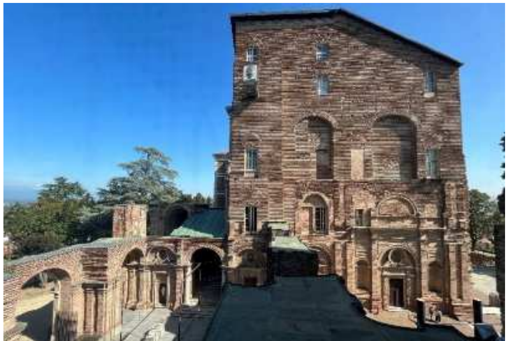
Fig. 5 - Juvarra's unfinished after A. Bruno's restoration. (CAL 2023)
