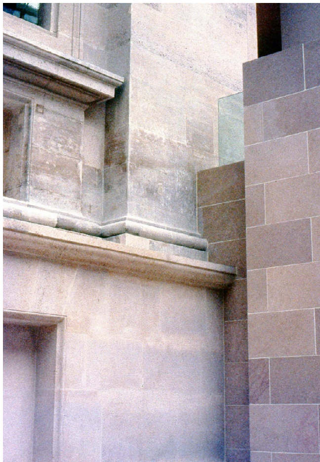
Fig. 46 - New constructions joining the old ones. (CB 1996)
