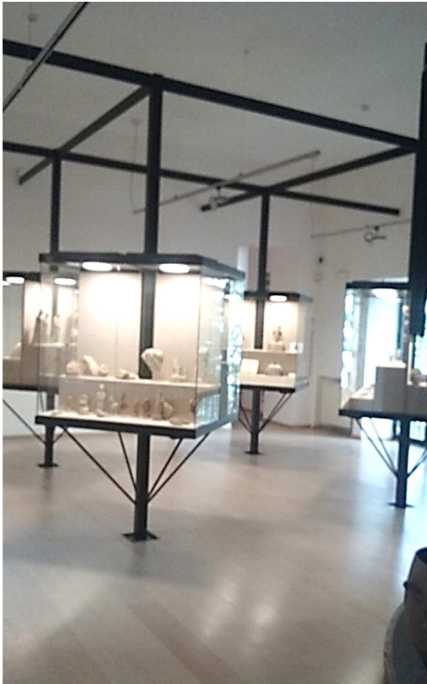
Fig. 73 - The system of modular show-cases hung from an aerial metal structure peripheral to each room allowed the entire floor area of each room to be left free for viewing, thus permitting the perception of spatial values. (CB 2021)
