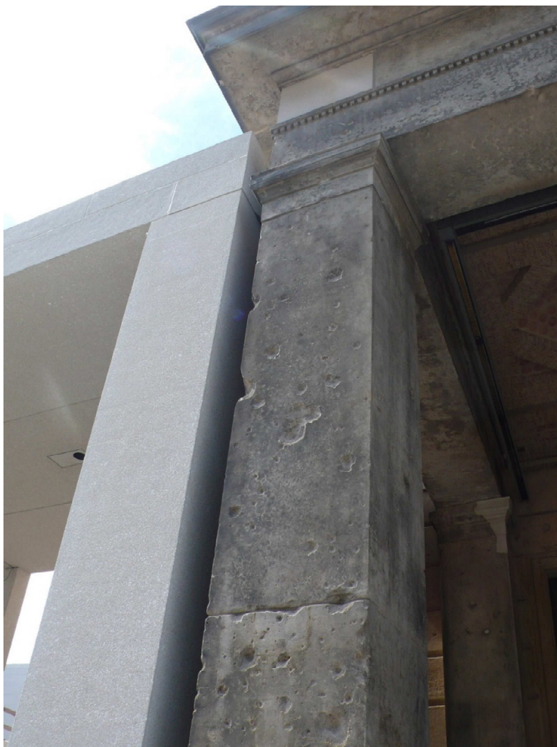
Fig. 40 - Detail of old and new columns. Traces of the War can be seen in the ancient pillar. (CB 2020)
