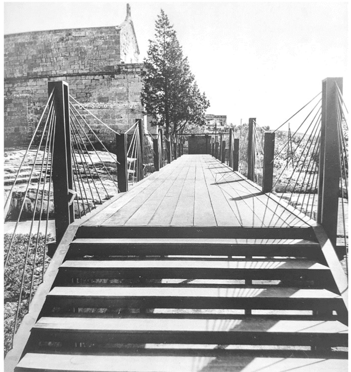
Fig. 37 - Detail of the walkway leading to the museum. Some construction details can be seen, such as the wooden beams and the slender column metal railings. (CB 1978)
