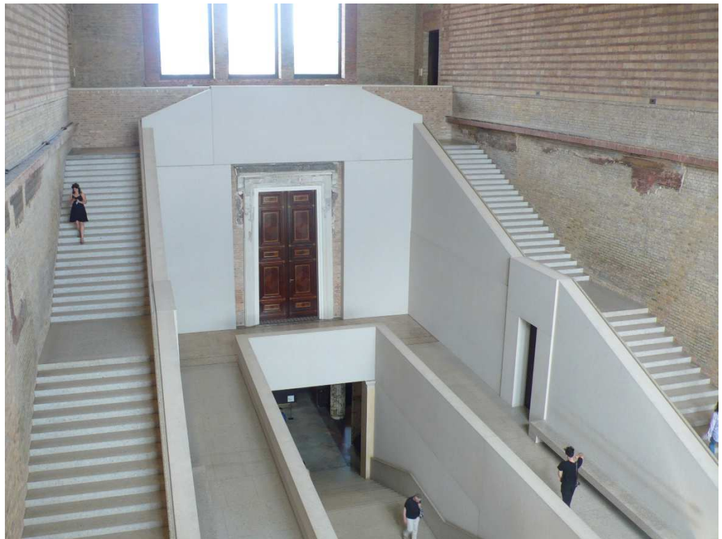
Fig. 17 - Stairhall. 2020 New construction of the stairs. The door is the only thing remained. (CB. 2020)
