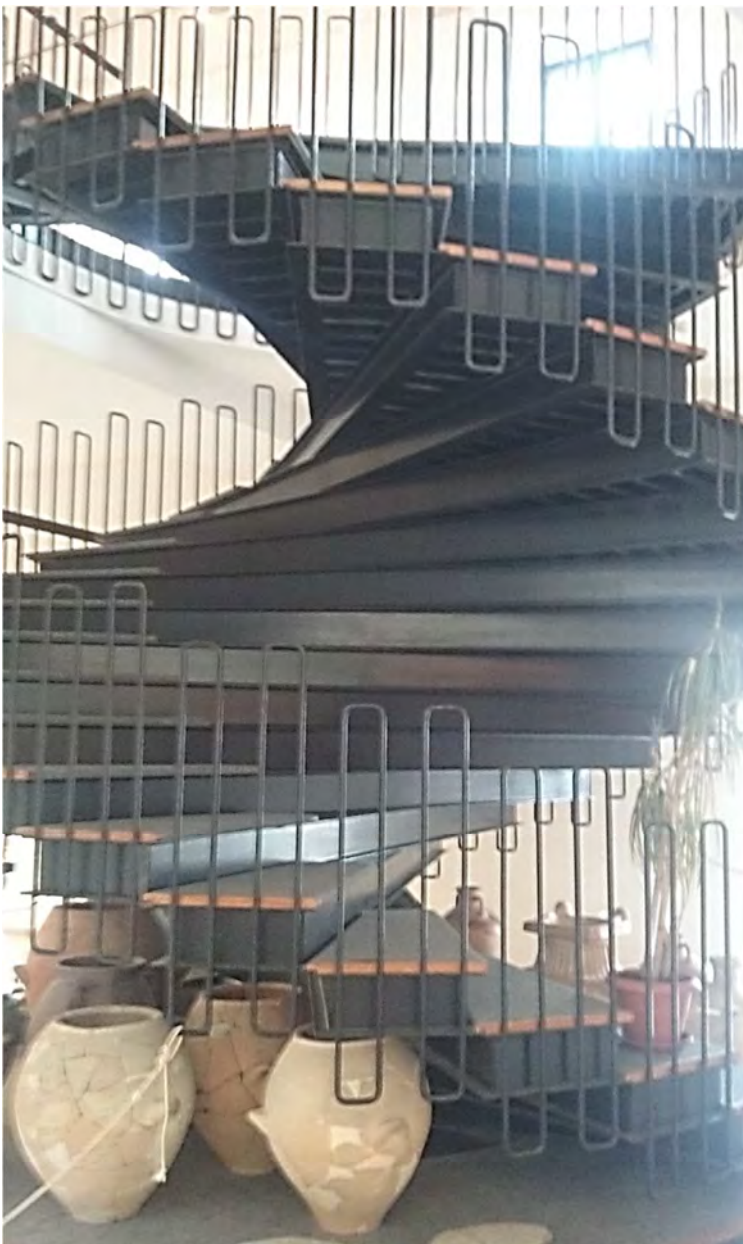
Figs. 78-79 - Detail of the stairs. The peculiarity is that on one hand you go up and, on the other different side, you go down. (CB 2021)
