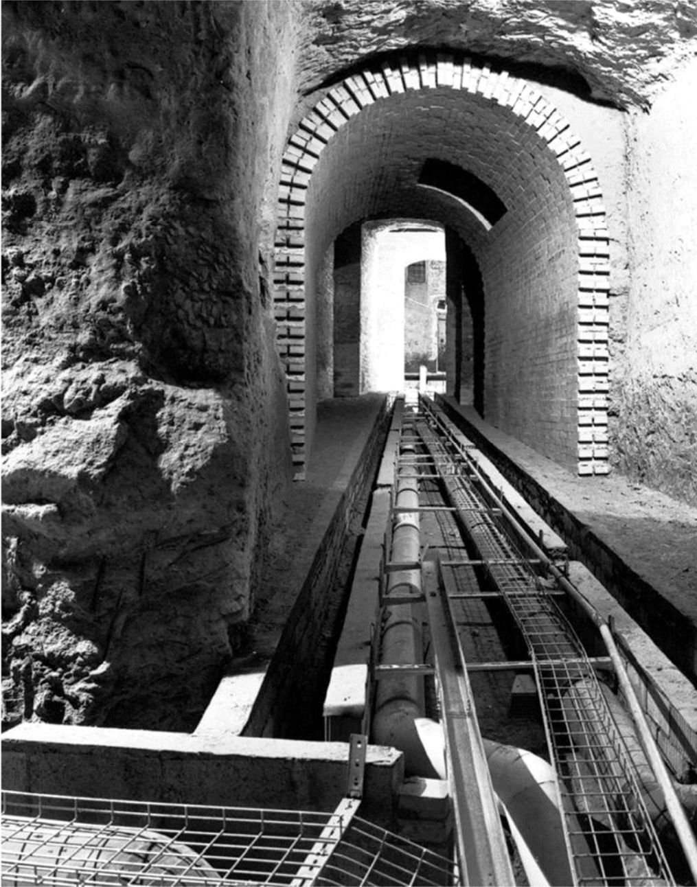
Fig. 21 - Work in progress on the installation of systems under the wooden platform. (From G. LONGOBARDI, Complesso museale Santa Maria della Scala , in "Musei, grandi tascabili architettura", Roma 2011, p. 22)
