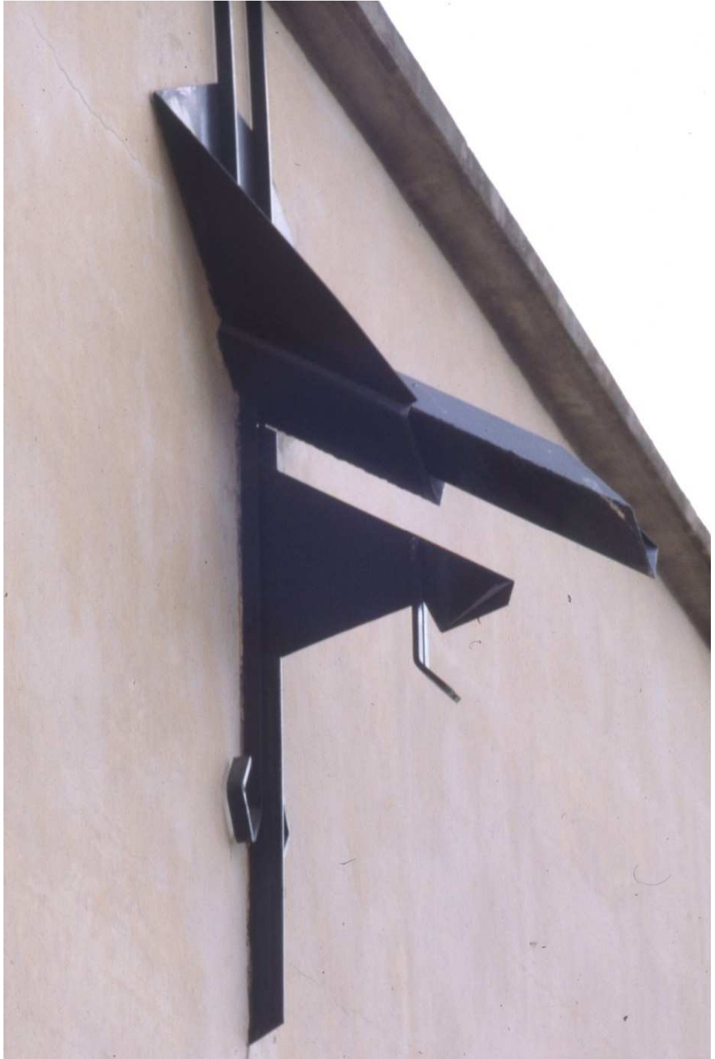
Fig. 5 - Particular for rainwater drainage in Agrigento. (CB 1982)
